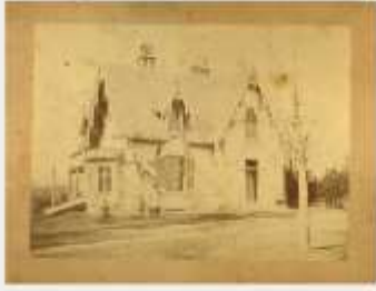
Five Oaks, before the tower was built, undated (Dayton Metro Library, FPW, Box 9, Folder 23)
